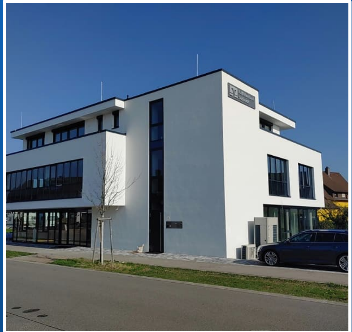
Sustainable branch of the Raiffeisenbank Südhardt eG with solar panel and e-charging station
